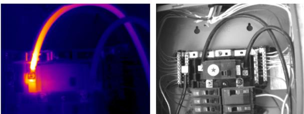
The photos above are of the same electrical panel. Comparing the two images, the fault can be clearly seen in the infrared photo but not to the naked eye. A hazard like this could shut your operation down or worse, cause a fire. Let our predictive services help you today!
